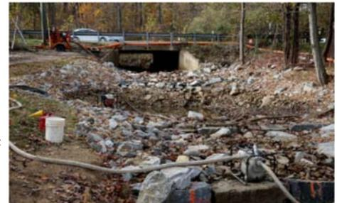
The project will include creek bank reinforcement with stones and matting along the creek edges made of coconut fibers that will keep soil out of the creek until vegetation becomes established.
